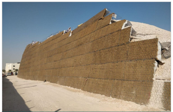
During construction: installation of Terramesh Green on outer steep slope
