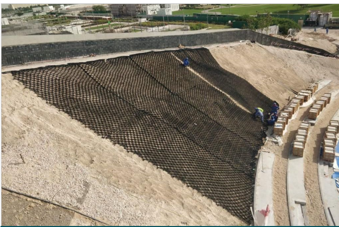
During construction: Laying of MacWeb geocell on inner gentle slope
