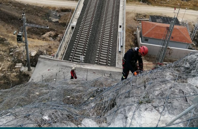
HEA PANEL INSTALLATION
