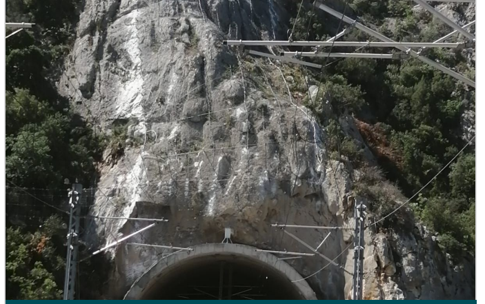
HEA PANEL INSTALLATION AT TUNNEL PORTAL
