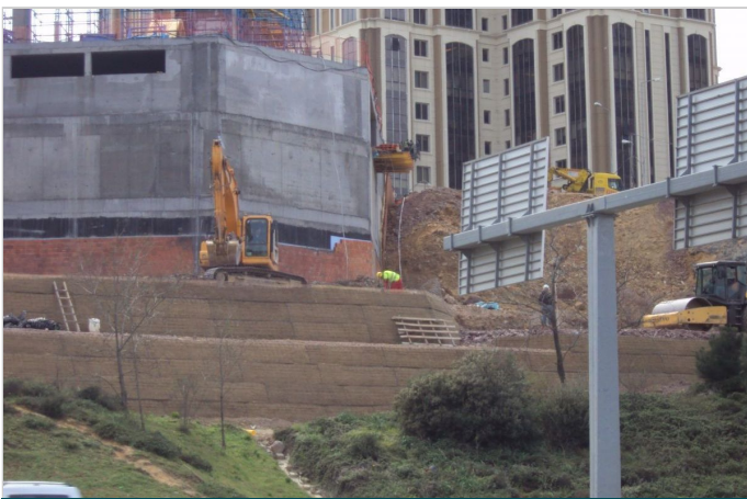
Green Terramesh Retaining Wall Construction Phase
