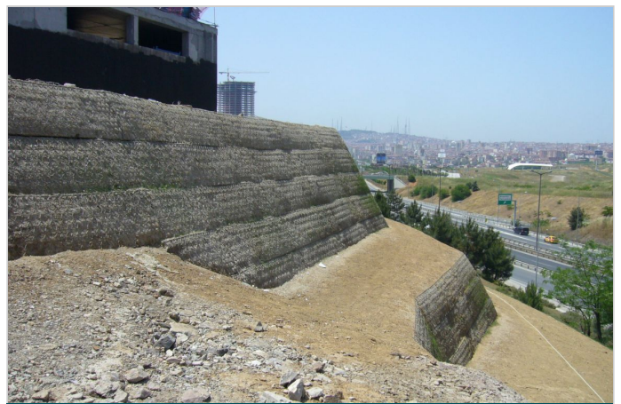
Green Terramesh Retaining Wall Construction Phase
