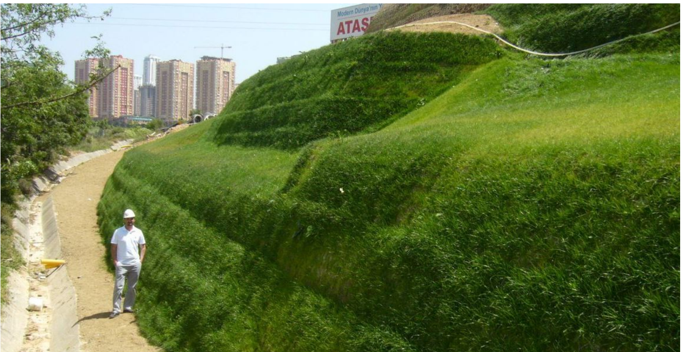
After The Completion of Green Terramesh Retaining Wall
