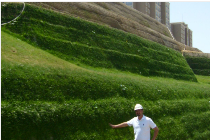
After The Completion of Green Terramesh Retaining Wall
