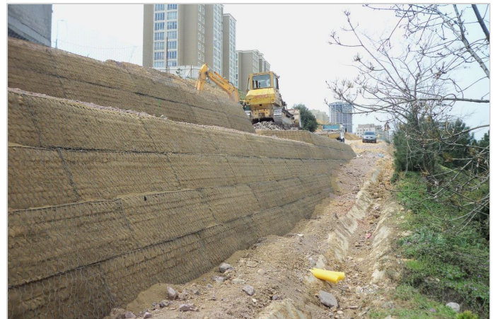
Green Terramesh Retaining Wall Construction Phase
