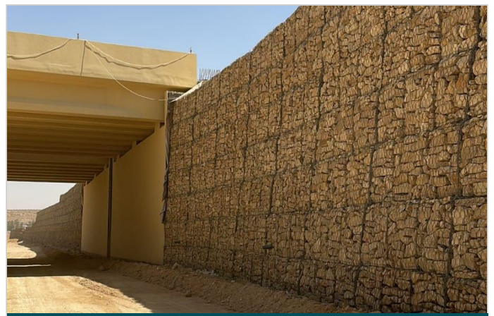
Ongoing Terramesh MSE wall
