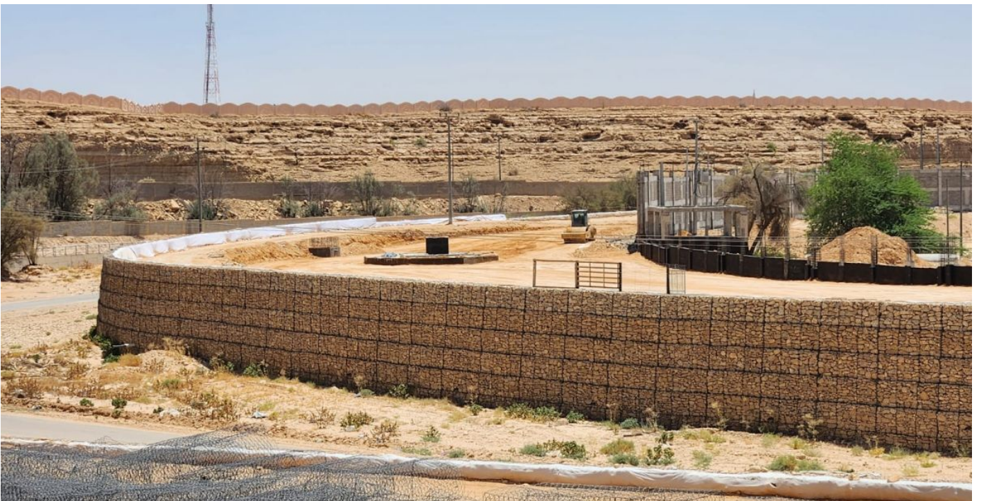
Ongoing Terramesh MSE wall along a long stretch
