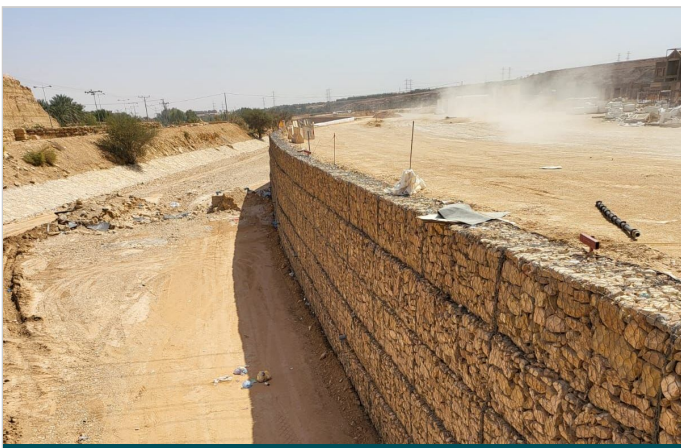
Ongoing Terramesh MSE wall
