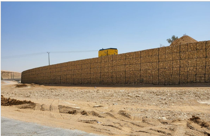
Ongoing Terramesh MSE wall
