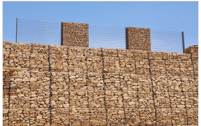
Weldmesh barrier above Terramesh MSE wall
