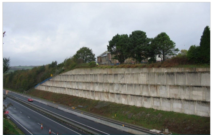
Retaining wall on a key route to the West country
