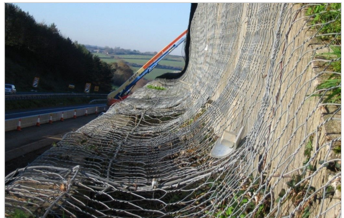
Steelgrid mesh anchored to the original slate
