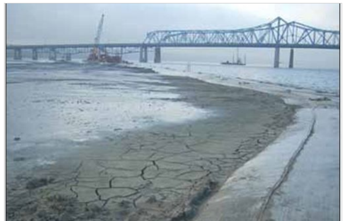
Backfilling the island after the perimeter was established
