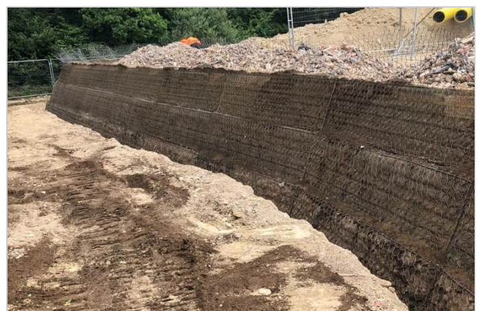
Structural backfill placement
