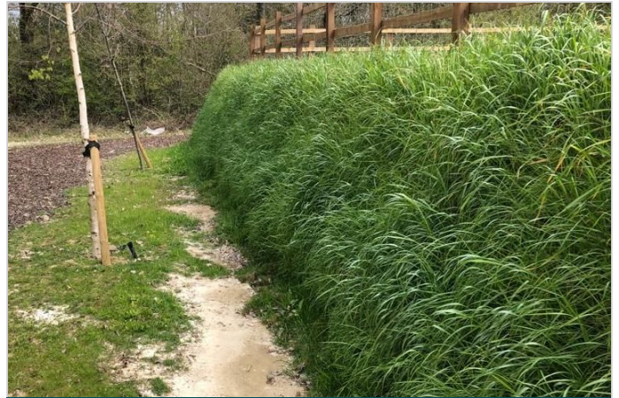
Green Terramesh slope - vegetation established
