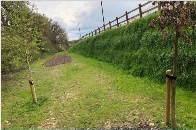
Green Terramesh slope - vegetation established
