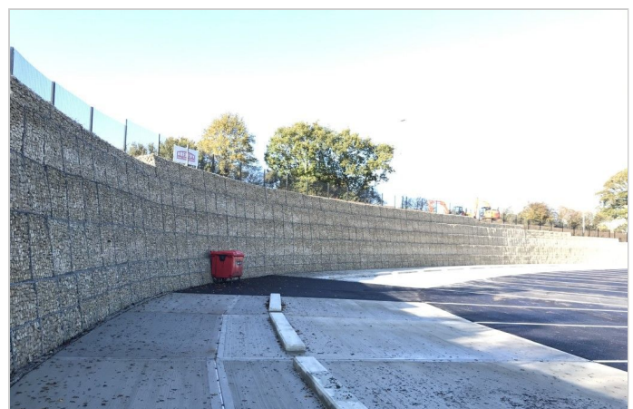
Neatly placed stone in the gabions minimising voids
