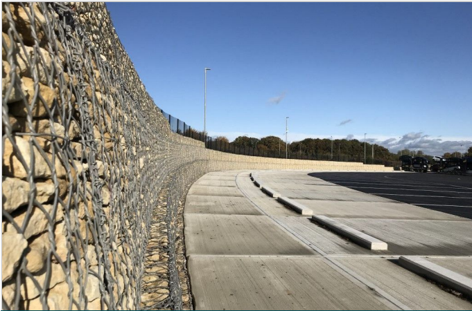
Terramesh® wall runs to edge of parking area and steps down
