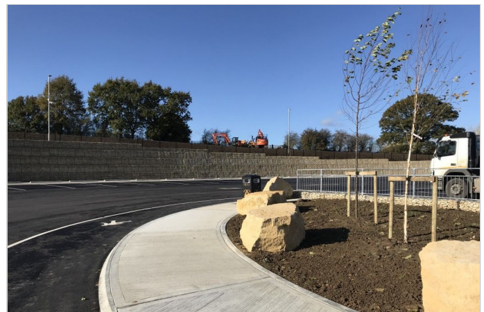
The tallest part of the wall at 5.5m high
