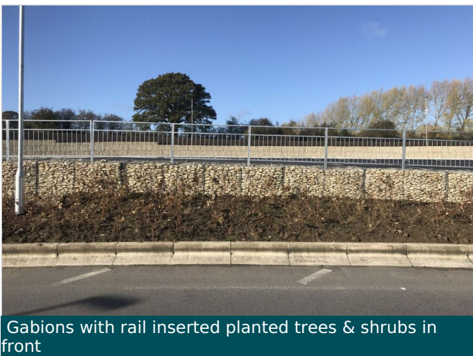
Terramesh® wall runs to edge of parking area and steps down
