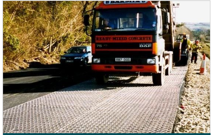
The paving operation continues
