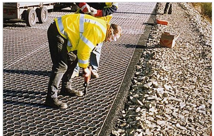
Locally fixing Road Mesh™ to the regulating layer
