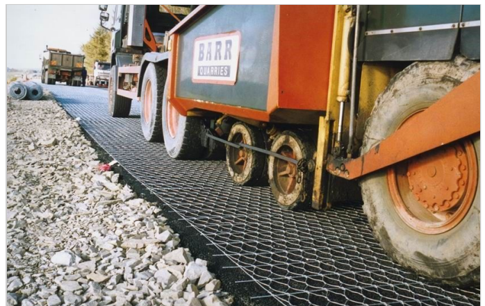
Close-up view of paving machine receiving asphalt
