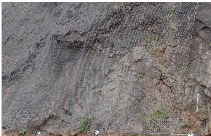
Steelgrid HR 100 PVC secured at the bottom of the slope
