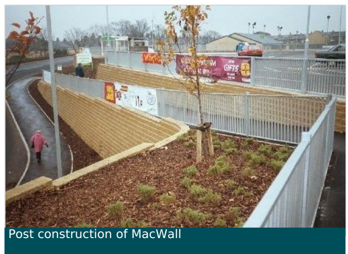
Post construction of MSE Wall
