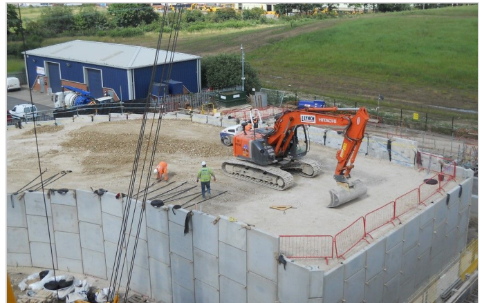
Construction taking place at EFW in North Hykeham
