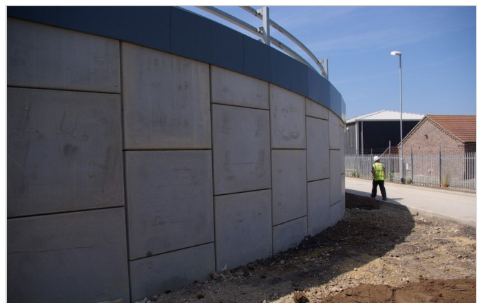
The completed structure at EFW North Hykeham
