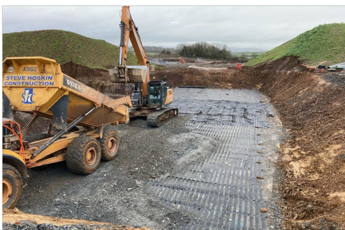
Backfill dumped and distributed onto ParaLink®
