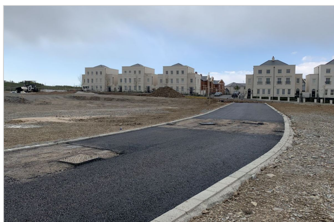
Estate roads construction on top of ParaLink® void spanning
