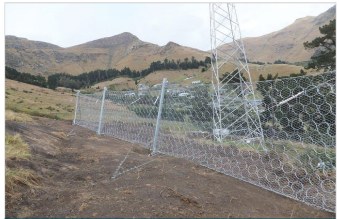
Complete Barrier Installation Works: Side View 2
