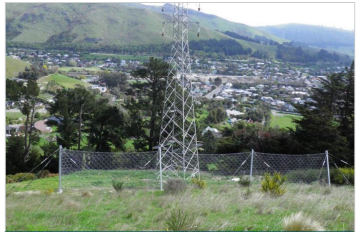
Complete Barrier Installation Works: View From Upslope
