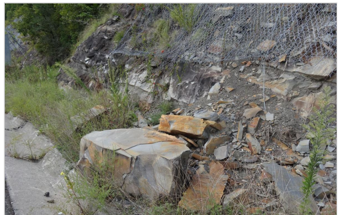
Blocks On the Toe of the Slope
