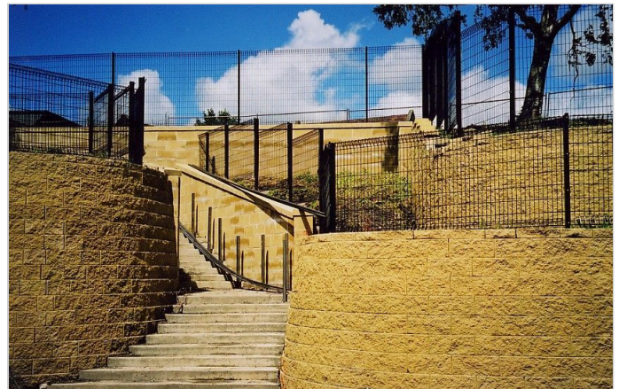
Post construction of MacWall
