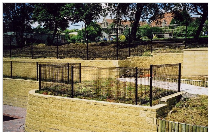
Post construction of MacWall
