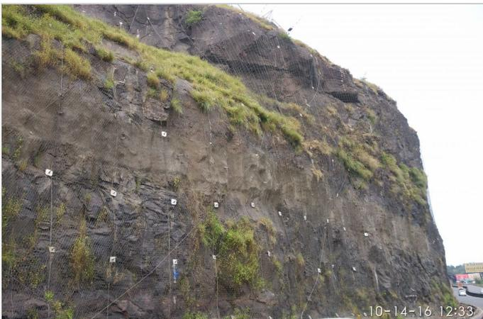
Figure 5-Shotcrete work, Steelgrid, HEA Panel and Diagonal Wire ropes installed
