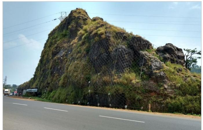
Figure 6-Completed Works- Cable Belting and Secured Drapery
