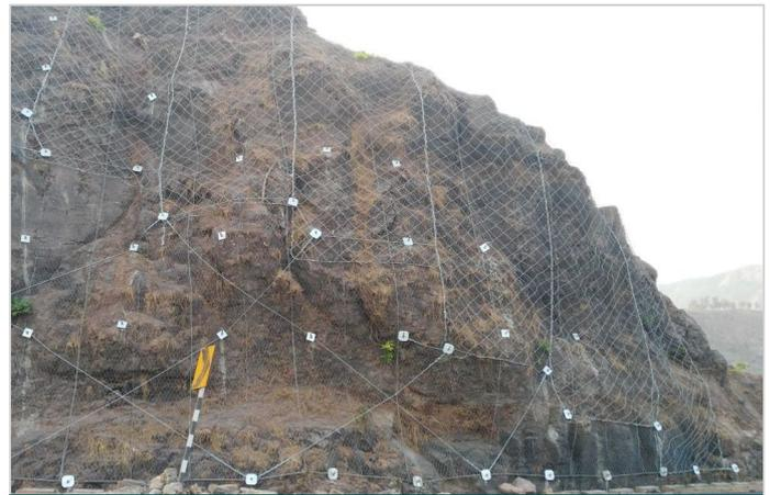
Figure 4-Steelgrid, HEA Panel and Diagonal Wire rope installation
