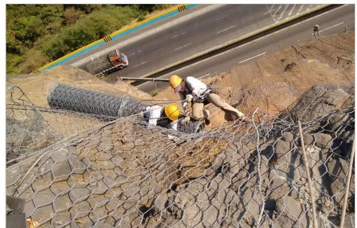
Figure 2-Steelgrid installation ongoing
