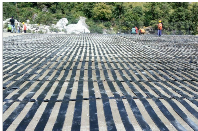
Photo 4: Laying of ParaLink
