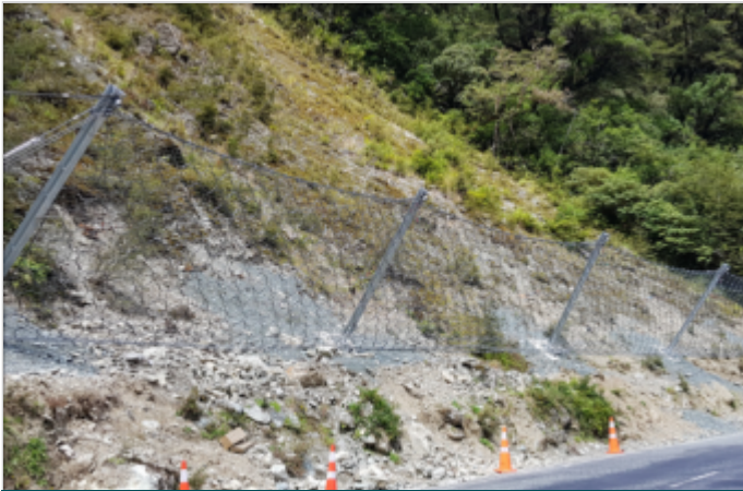
Completed 2000 kj Maccaferri RMC200A certified fence
