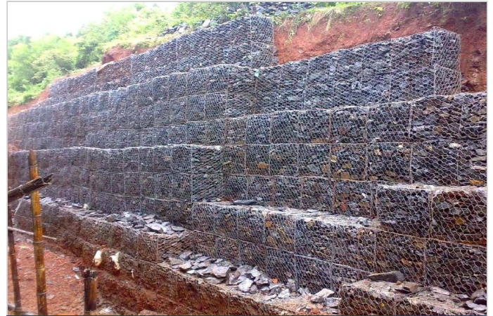
Photo 4: Photograph showing the gabion boxes filled with stones
