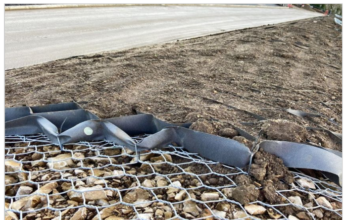
MacWeb® and DT Mesh Installation
