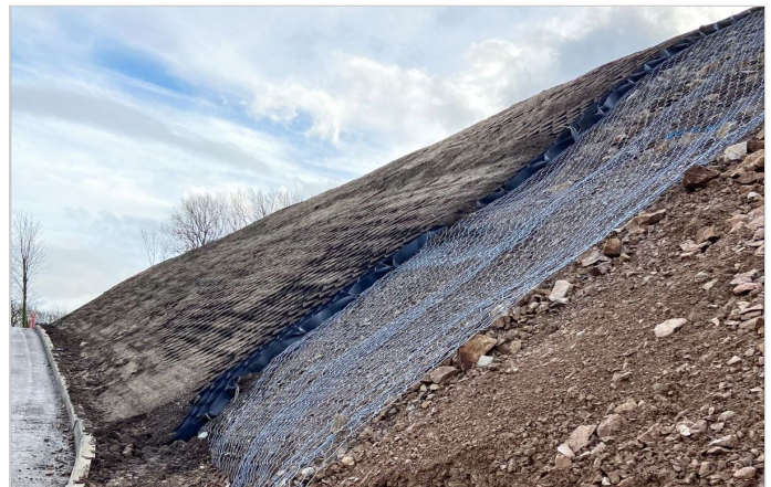
Slope at 45° with MacWeb® and DT Mesh Installed
