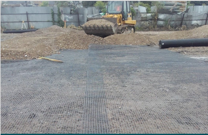
MacGrid EG40S laid with min 300mm roll overlap
