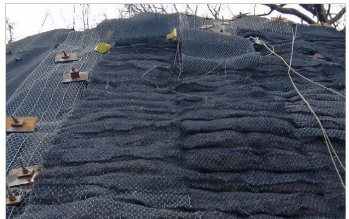
Vegetative soil wrapped on MacMat® R.
