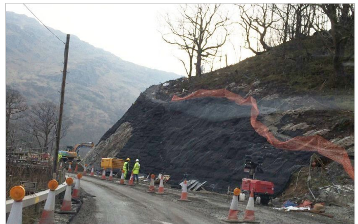
View of the rock cutting slope at initial stages.
