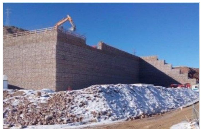
Crusher Terramesh System Retaining Wall
