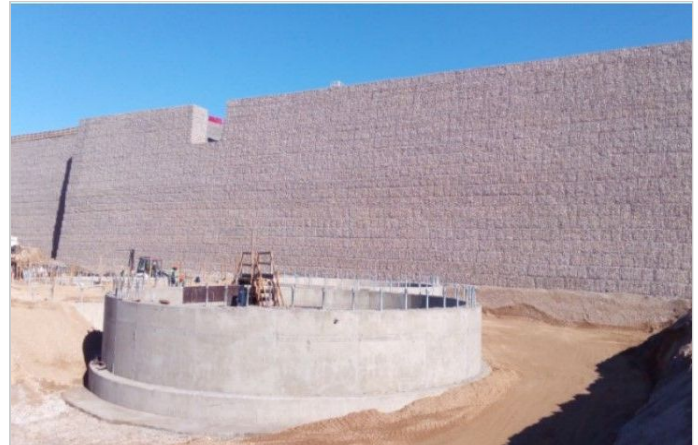
Grinder Terramesh System Retaining Wall
