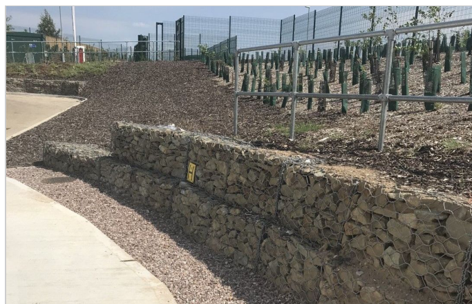
Gabion retaining wall
