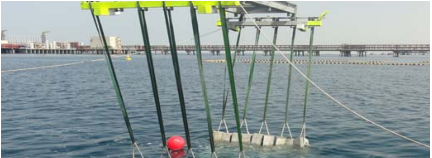
TAKREER CARBON BLACK & DELAYED COKER PROJECT
