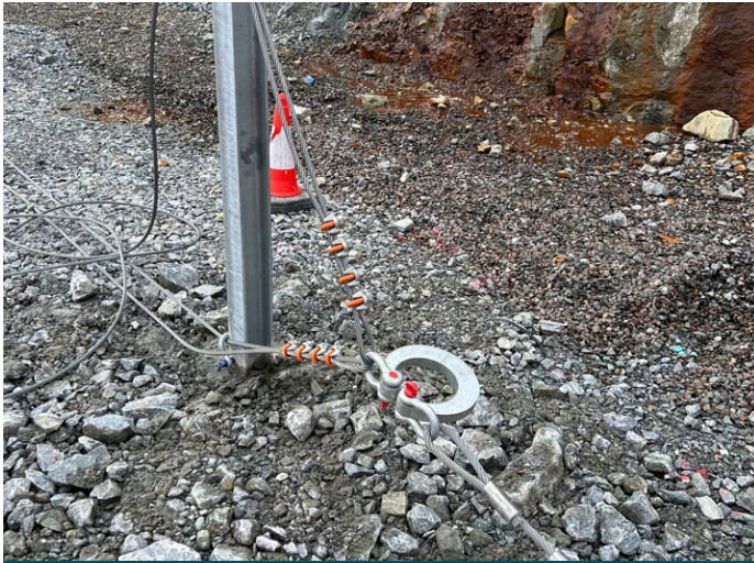
Energy dissipating device connected to lateral anchor
