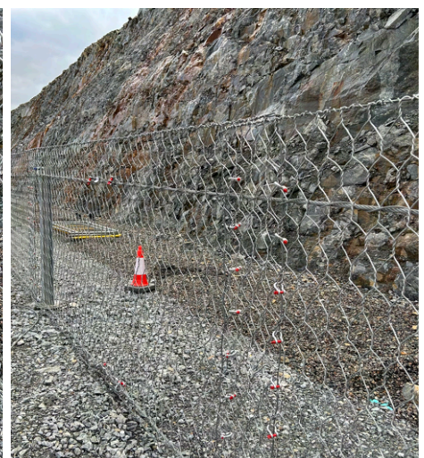
Fully constructed RB35 NP 1.35m high
