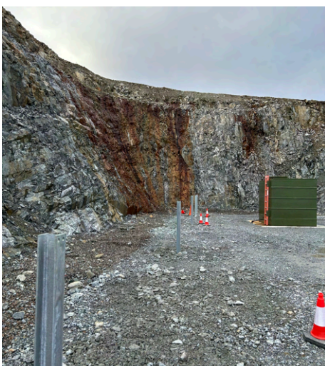
RB35 NP (no plate) 1.35m high posts set
