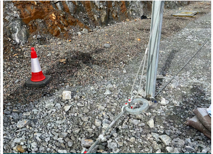
Energy dissipating device connected to lateral anchor
