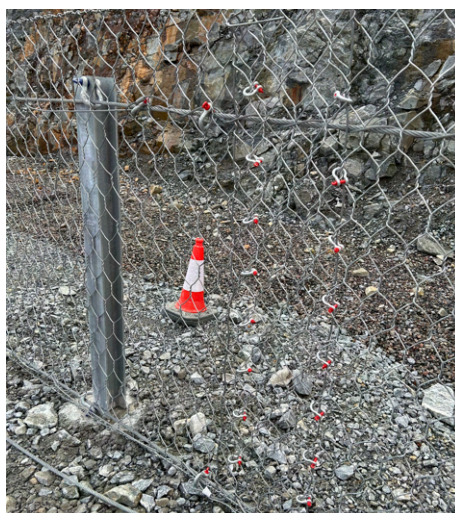
Double twist interceptor mesh connected
