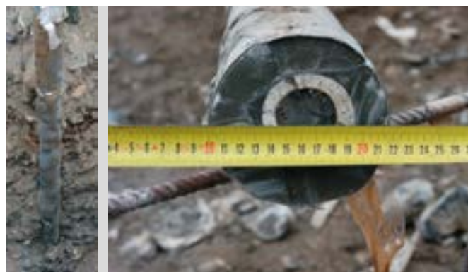
Expansion of a P.E.R. Ground (R) bar after injection
