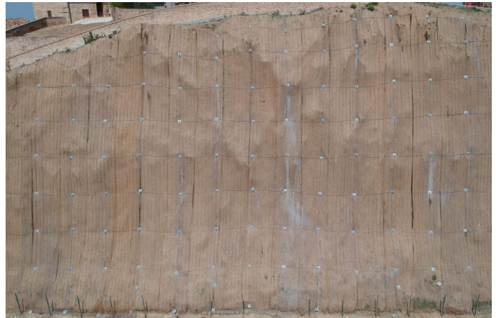
Detail of the works
