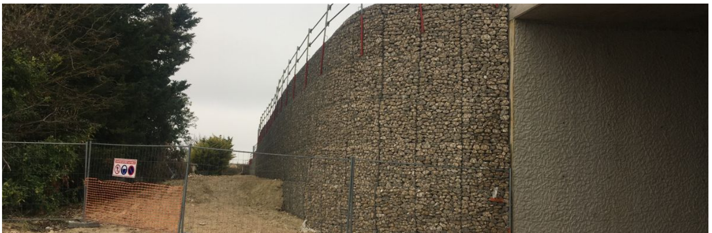
Terramesh System wall
