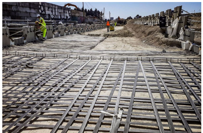
ParaWeb Abutment C1
