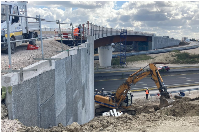
Abutment C1 & C3
