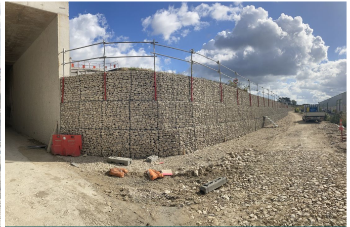
Terramesh System wall
