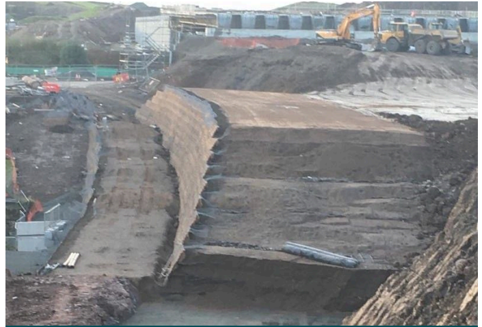
GTM and Paragrid. The structure is getting higher
