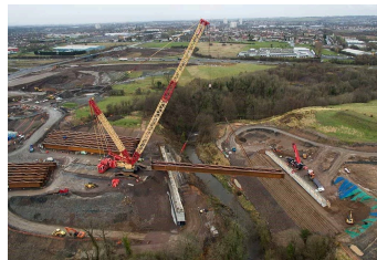
The North Calder bridge beam
