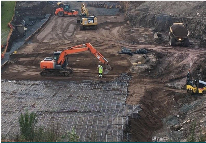
Paragrid geogrid placed in layers as designed by Amey/RPS
