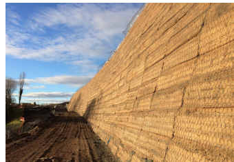
Finished 15 metre high slope
