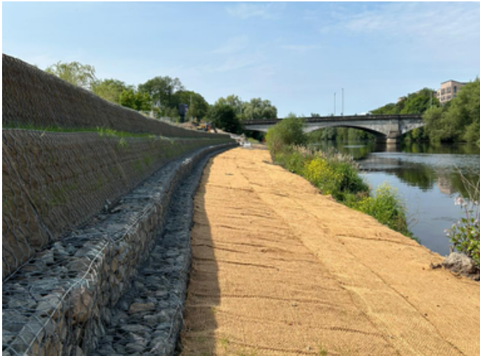
Riverbank restoration with Green & Gabion Terramesh with erosion
