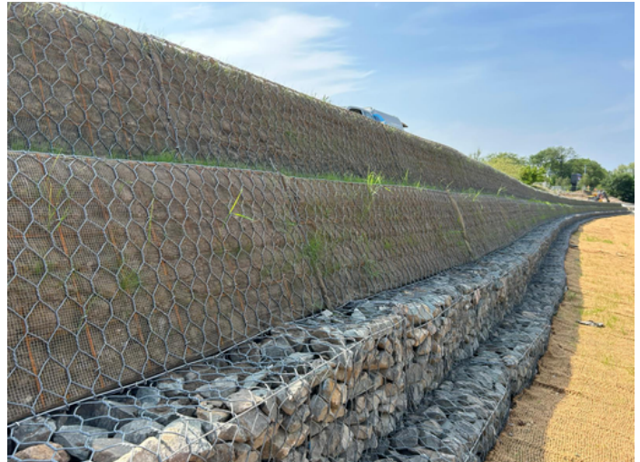
Close up detail of Green & Terramesh systems embankment
