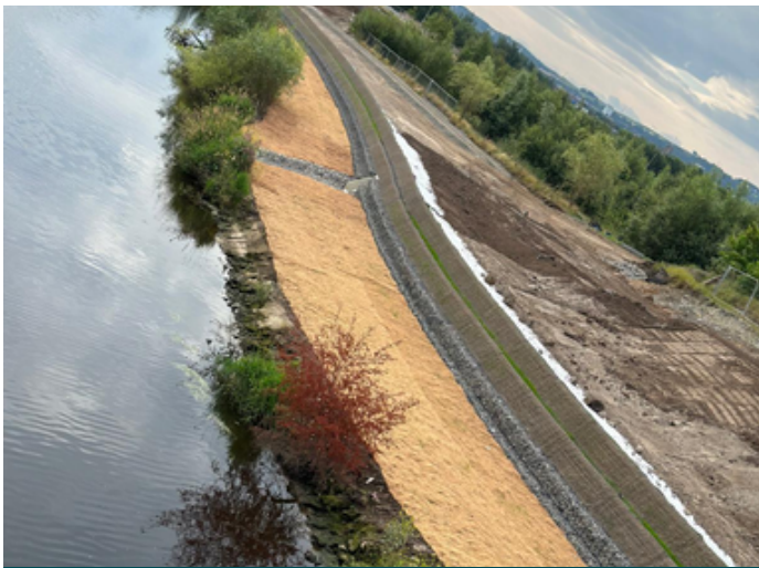
View of completed works
