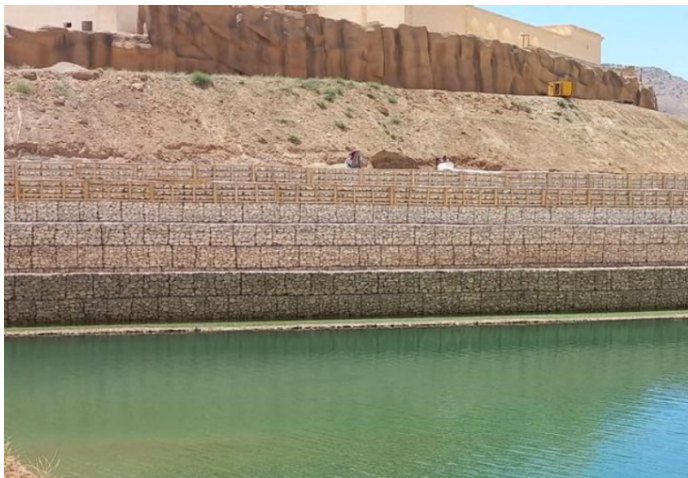
During Construction—After Rising of Water Level
