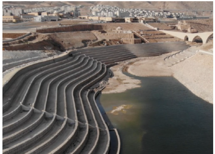
Terramesh System Walls
