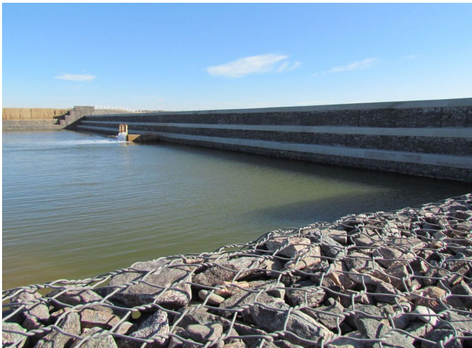
After the construction
