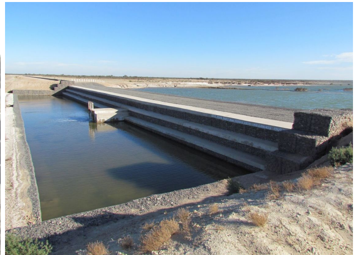
After the construction
