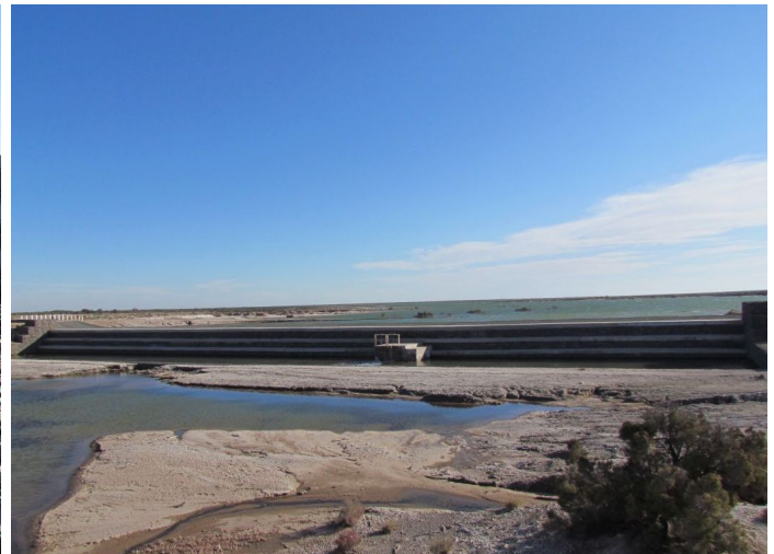
After the construction
