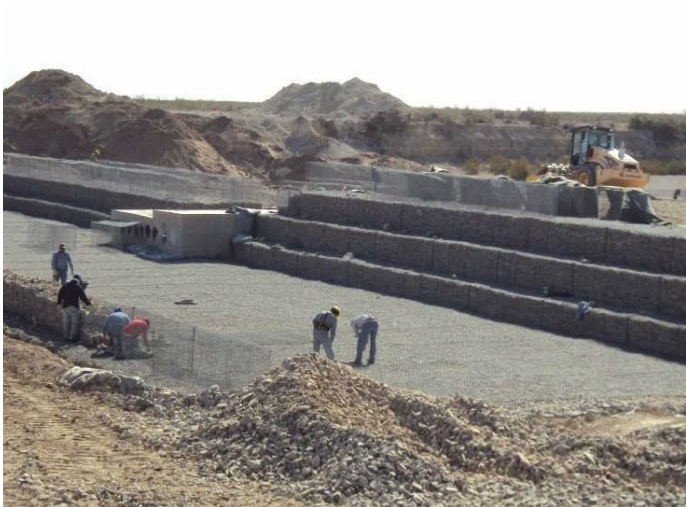
During the construction
