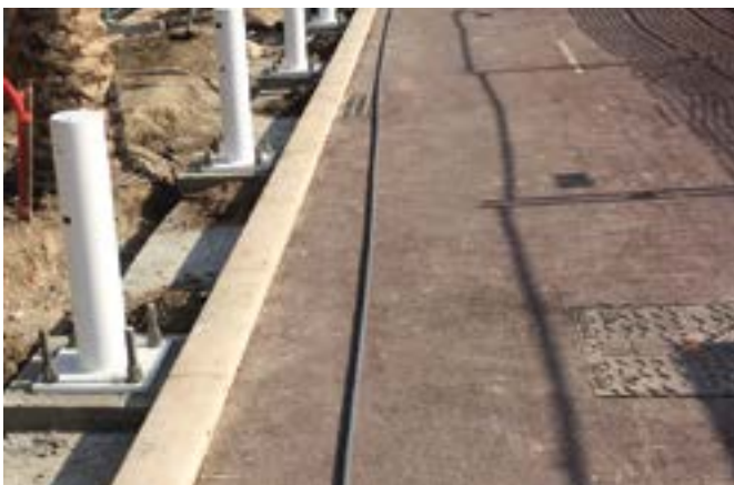
Fixing posts to ground foundations
