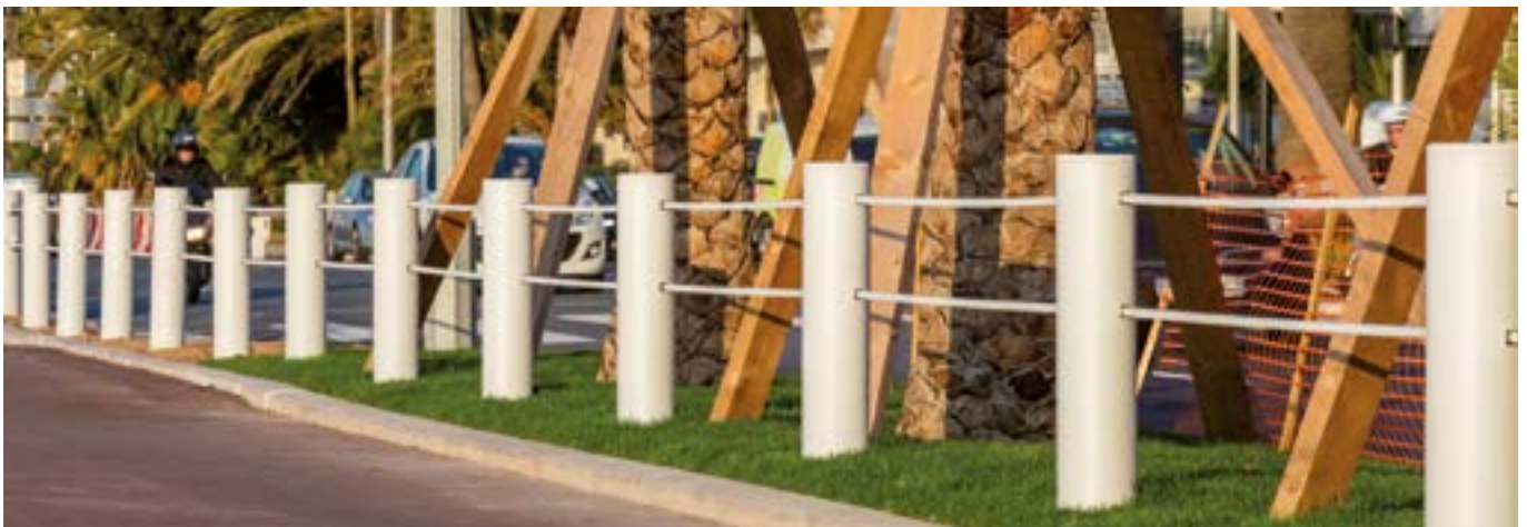
MacSafe® completed installation adjacent to pedestrian zone
