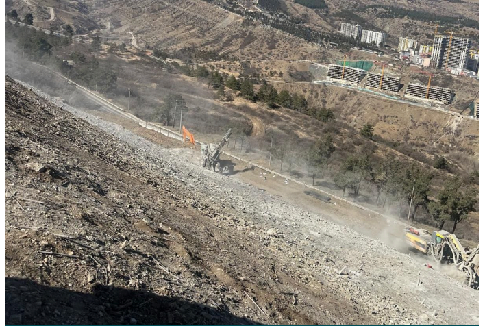
Pre-Installation Condition of the Slope
