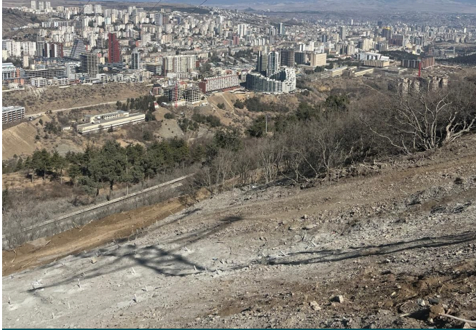
Pre-Installation Condition of the Slope
