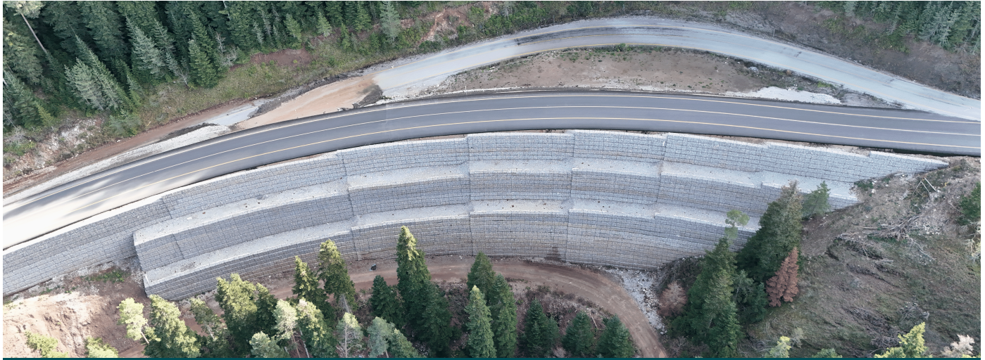
After Construction Phase
