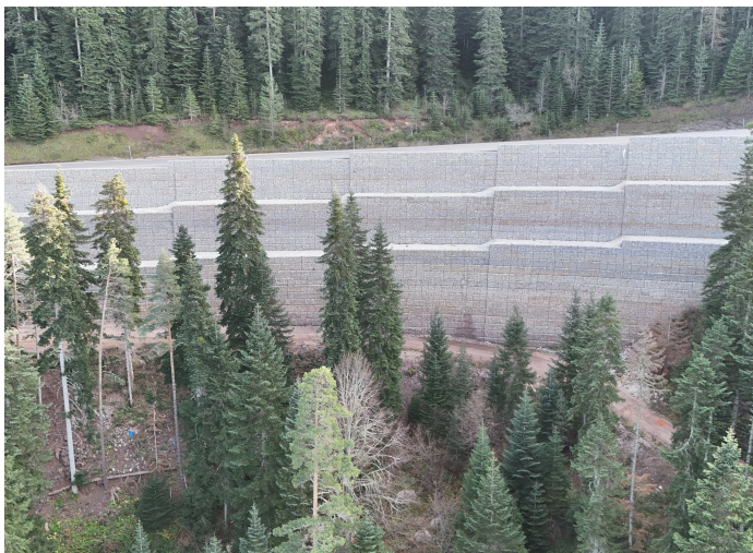
After Construction Phase
