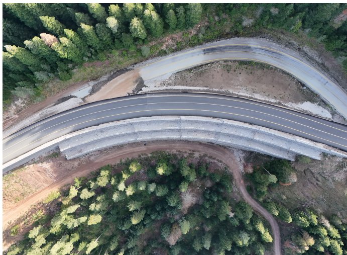
Terramesh Wall From Above
