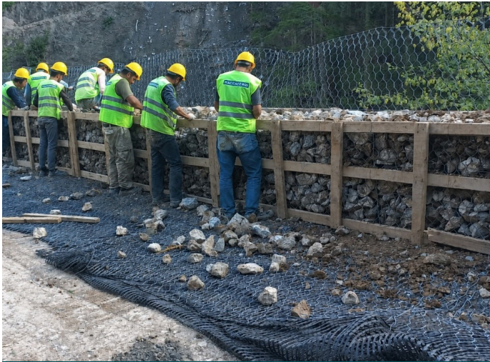
During Construction Phase
