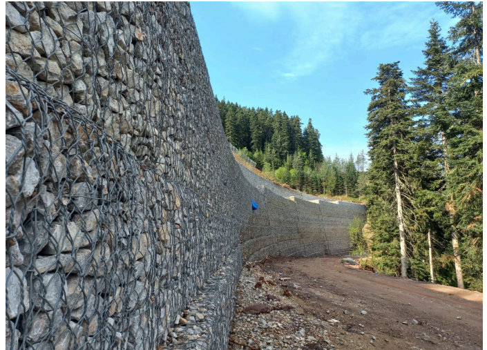
The Front of the Terramesh Wall
