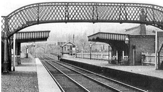
St. Ann's Well Station
