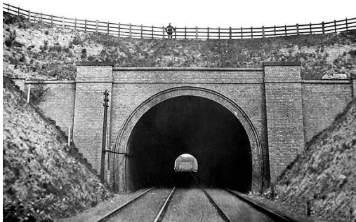
Sneinton Tunnel South
