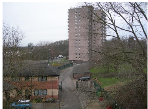
2007: Woodthorpe and Winchester Court Flats
