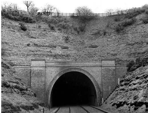
Sherwood Tunnel South
