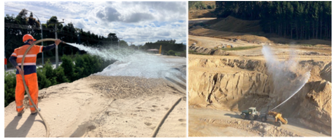
Polymer being applied to a pumice stockpile to prevent dust and water carts using cannons in action to manage dust over big spaces.
