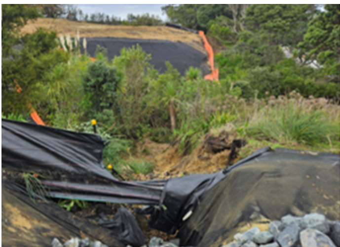
Damage to pond outlet and bank below SRP post storm event
