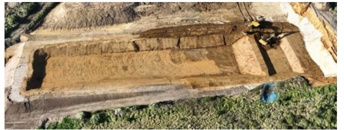
Pond constructed in pumice soils being ash and clay lined.
