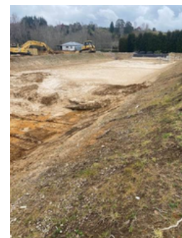
Pond constructed in pumice soils being ash and clay lined.
