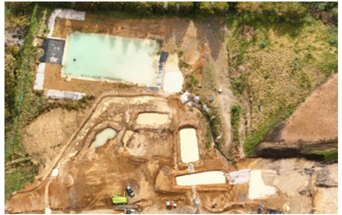
Pre-forebay forebays prior to SRPs to help slow water down and encourage sediment drop out prior to the Sediment Retention Device.
