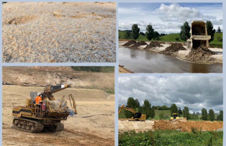
Photos: Top and bottom left showing some hydro mulch applied to pumice surface to help reduce rainfall erosion. Top and bottom right showing pumice soils being encapsulated with topsoil or ash/clay to prevent erosion.
