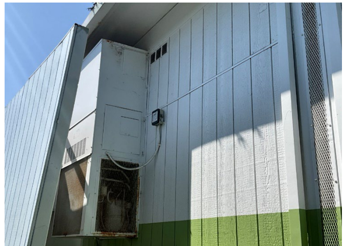
6 – WALL MOUNTED HEAT PUMP
