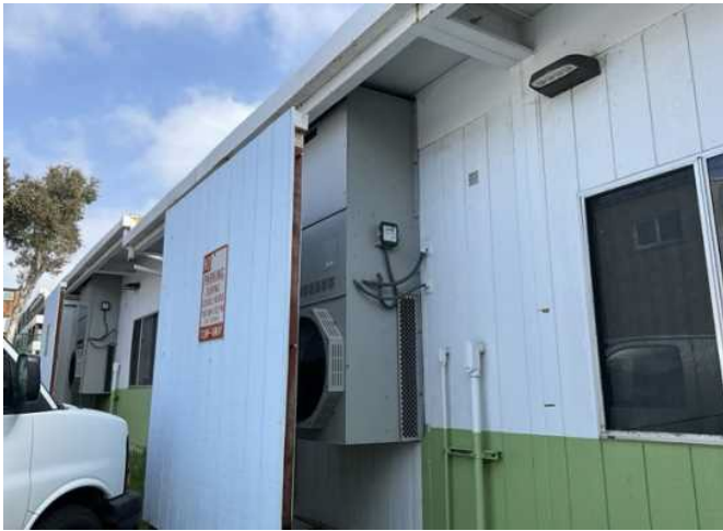
3 – WALL MOUNTED HEAT PUMP
