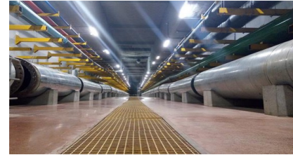
Underground Utility Tunnel
