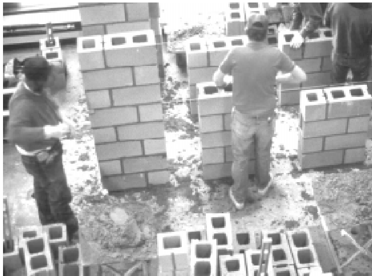
Figure 3—Construction of Specimens
