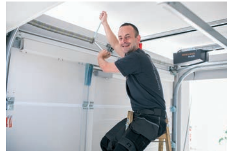
SECTIONAL GARAGE DOOR SPRING TIGHTENING
