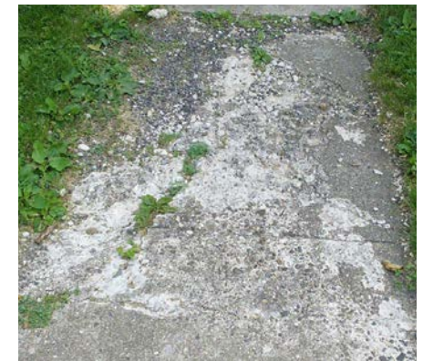
Surface Condition: Spalling
