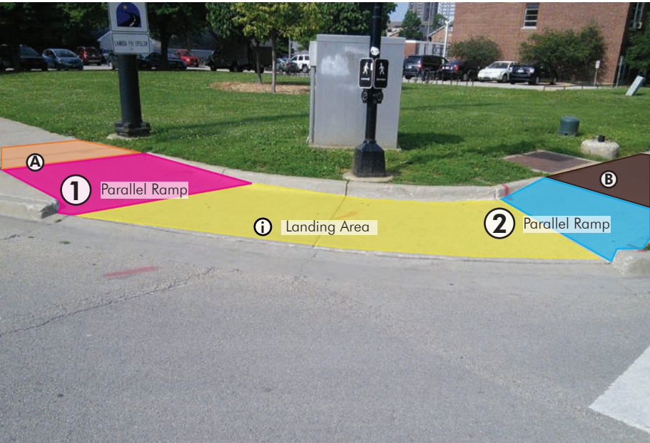
Figure A-7 Approaches for Parallel Ramps
