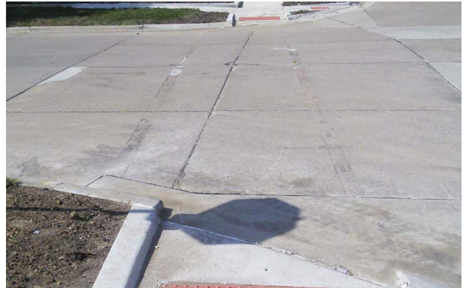
In this crosswalk, the standard painted markings and the stop bar are worn, almost to the point of being unrecognizable.
