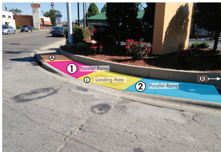
Figure A-8 Facing Parallel Ramps with a Detectable Warning Surface
