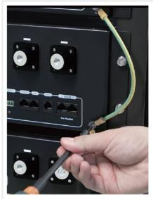
② Use the 2AWG 200mm battery parallel wires included in the packaging to connect the batteries in parallel.
