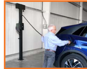
Auto-retracting cable management prevents harm to EV charger cables
