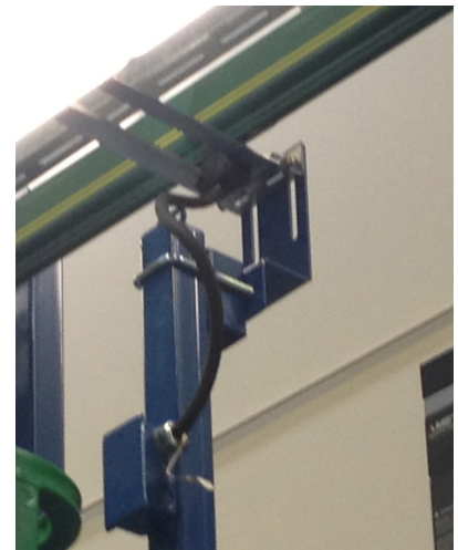
Proper alignment of Vahle energy rail and trolley
