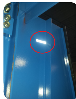
Reflective tape installed on outer frame panel
