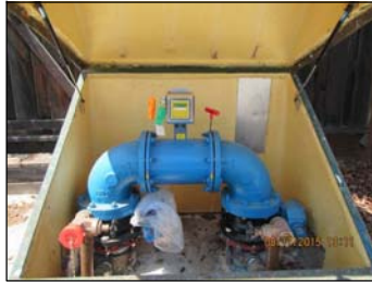
6-INCH CALWATER INTERTIE MARINE VIEW AVE
