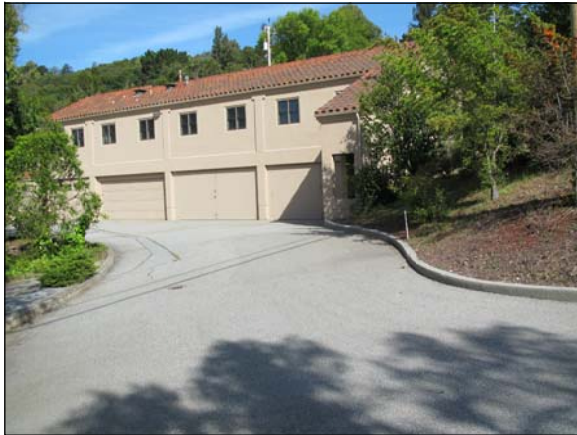
EXISTING MAINTENANCE BUILDING
