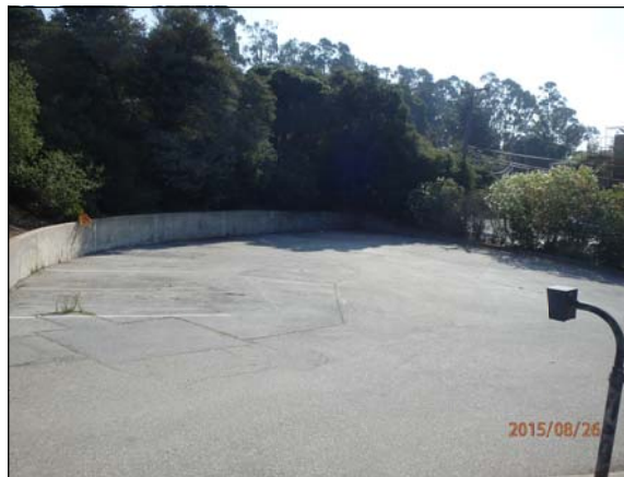
EXISTING PARKING LOT
