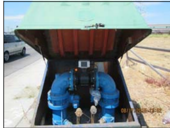
6-INCH CALWATER / REDWOOD CITY INTERTIE SHOREWAY RD
