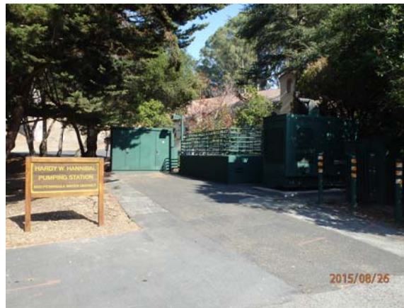
HANNIBAL PUMP STATION
