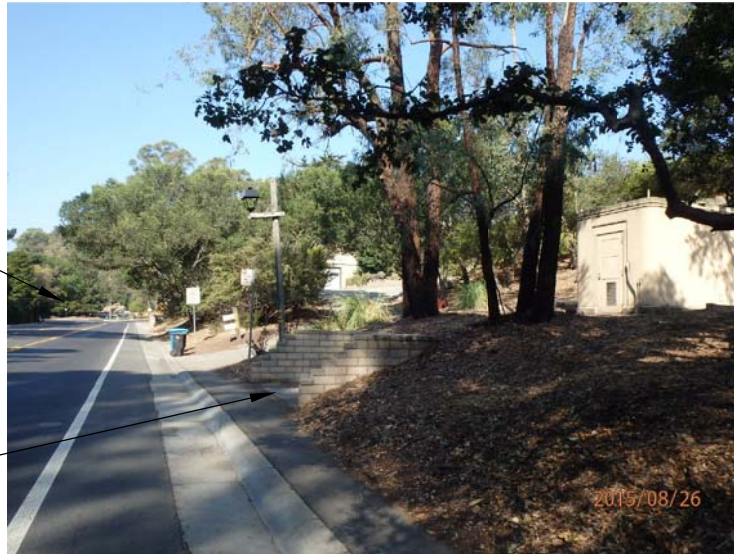
HANNIBAL PUMP STATION 600 FT WEST
