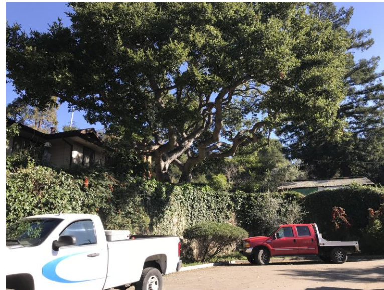
Perimeter Wall towards Adjacent Property
